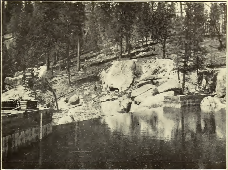
FIG. 1.—BULKHEADS AND CREST OF SPILLWAY, FROM UPSTREAM SIDE, LYONS DAM, CAL.
